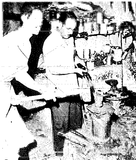
Figure 71 An Anvil Placed on a Wooden Block
