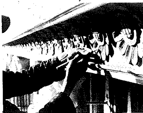
Figure 211 The Carving of Stucco Plaster
