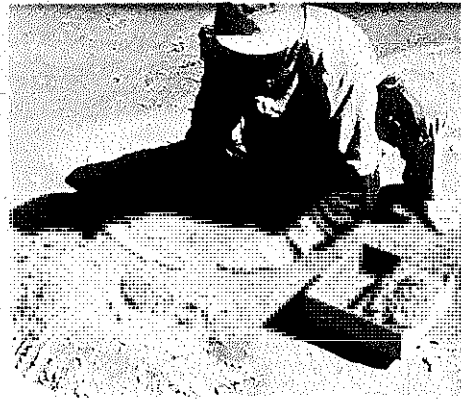
Figure 172 Filling the Brick Mold
