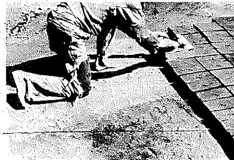
Figure 173 Emptying the Brick Mold
