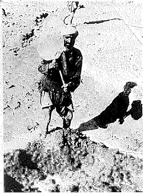
Figure 162 Preparing the Loam for Mud Bricks
