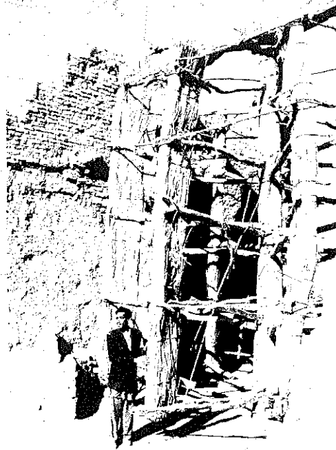
Figure 404 The Wind Wheel of the Sistani Mill
