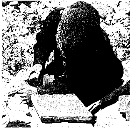
Figure 188 Grinding the Tile Edge
