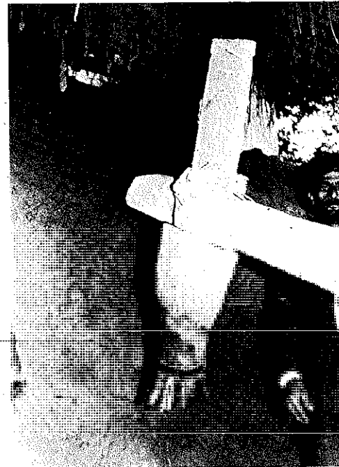
Figure 408 The Pestle of a Rice-Husking Mill
