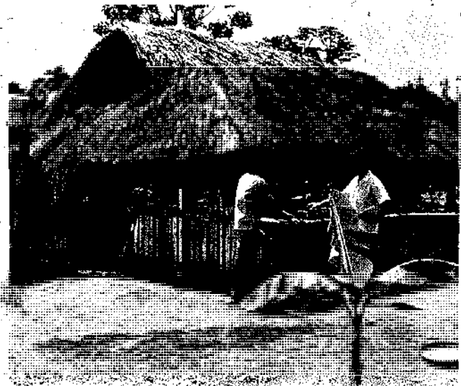
Pig house built of bush materials, Martyrs' High School, NP
