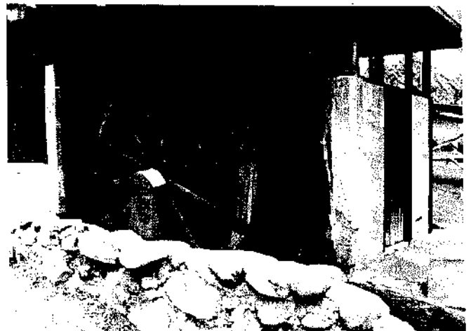
Overshot water wheel (above) and generator (below) at the Swiss Mission near Minj, WHP. Power is transmitted through a counter shaft in order to increase the rpm's.
