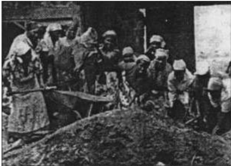
Mothers and grandmothers work together to build a cooperative bakery. Here they make mud bricks of earth mixed with straw.
