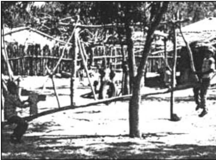
A teeter-totter (see-saw) in the crotch of a mango tree has a donkey on one end. The other end has an enclosed seat, with space behind it where a non-disabled child can sit and help support the disabled child.
