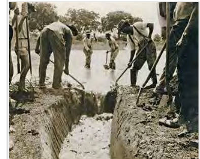
A 1920s photograph of efforts to disperse standing water and thus decrease mosquito populations
