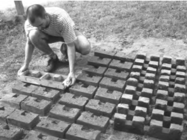
15-6 Production of special adobes
