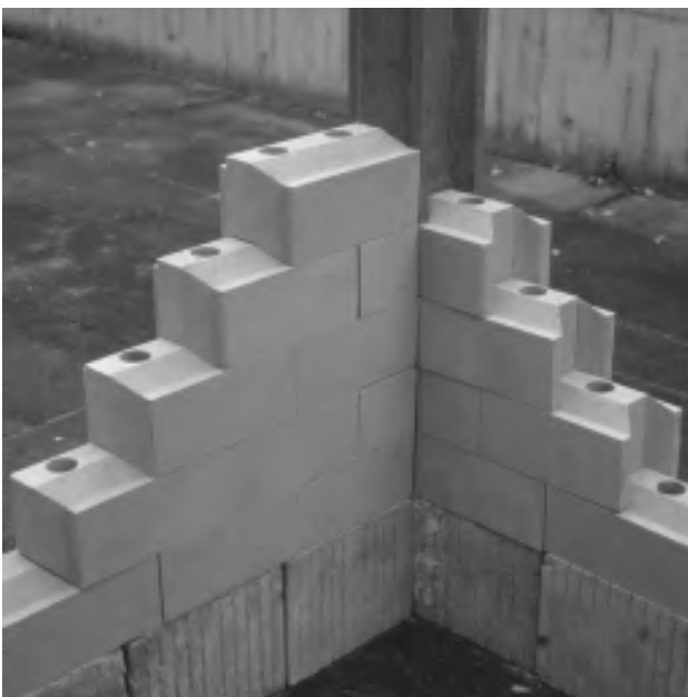
7-15 Improved interlocking system of FEB, Kassel, 2001
