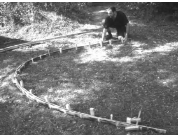
15-7 Construction of the arc with split bamboo
