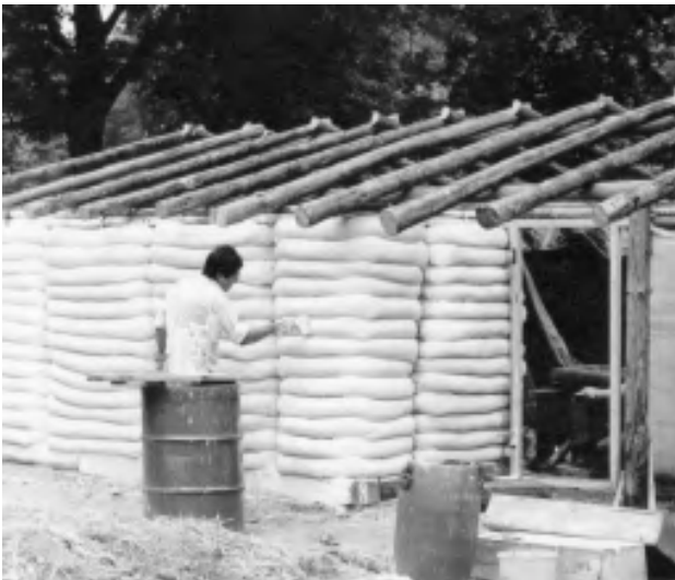
9-2 and 9-3 Wall with filled textile hoses
