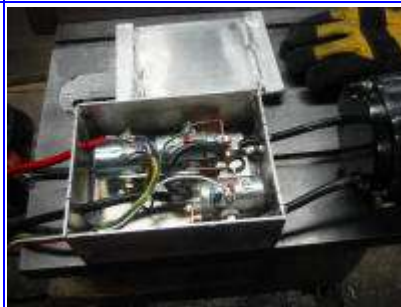
(4) Winch power relay box.
