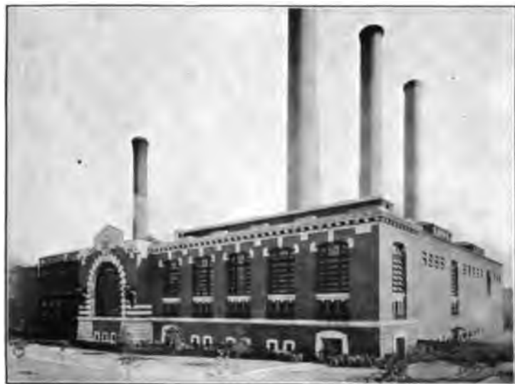
FIG. 287. — A modern power plant, the Edison power station at South Boston.
