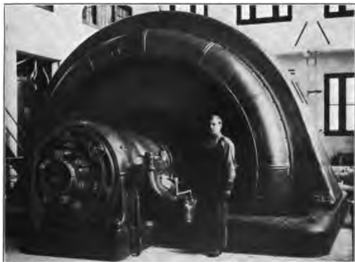
FIG. 280. — Synchronous condenser in substation at Eagle Rock, California, used to improve power factor on a very long transmission line. The exciter is in the foreground.
