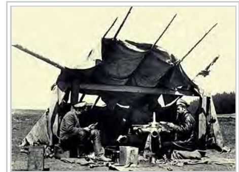
Field repair of aircraft engine (1915-1916 yy)
