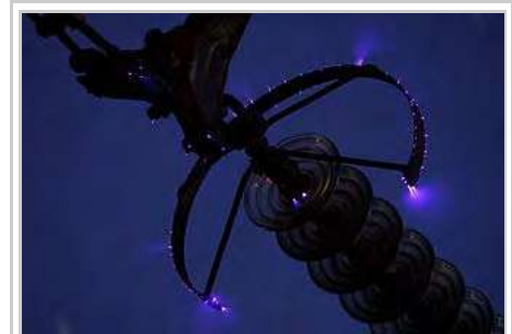
Long exposure photograph of corona discharge on an insulator string of a 500 kV overhead power line. Corona discharges represent a significant power loss for electric utilities.
