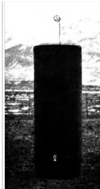
Tesla coil in one experiment of many conducted in Colorado Springs. This is a grounded tuned coil in resonance with a nearby transmitter; Light is glowing near the bottom.
