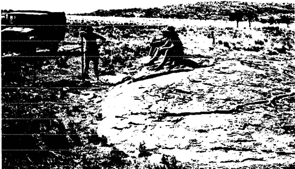
WEMIKUTTA. SMALL DOME FITTED WITH A CONCRETE GUTTER BY ANDREW AND KIM LEADS TO A NETTED TREE ENCLOSURE WITH PISTACHIO. (SEE FIG. 55). GUTTER IS SNAKE-LIKE LINE ON STONE. PLATE 5-7
