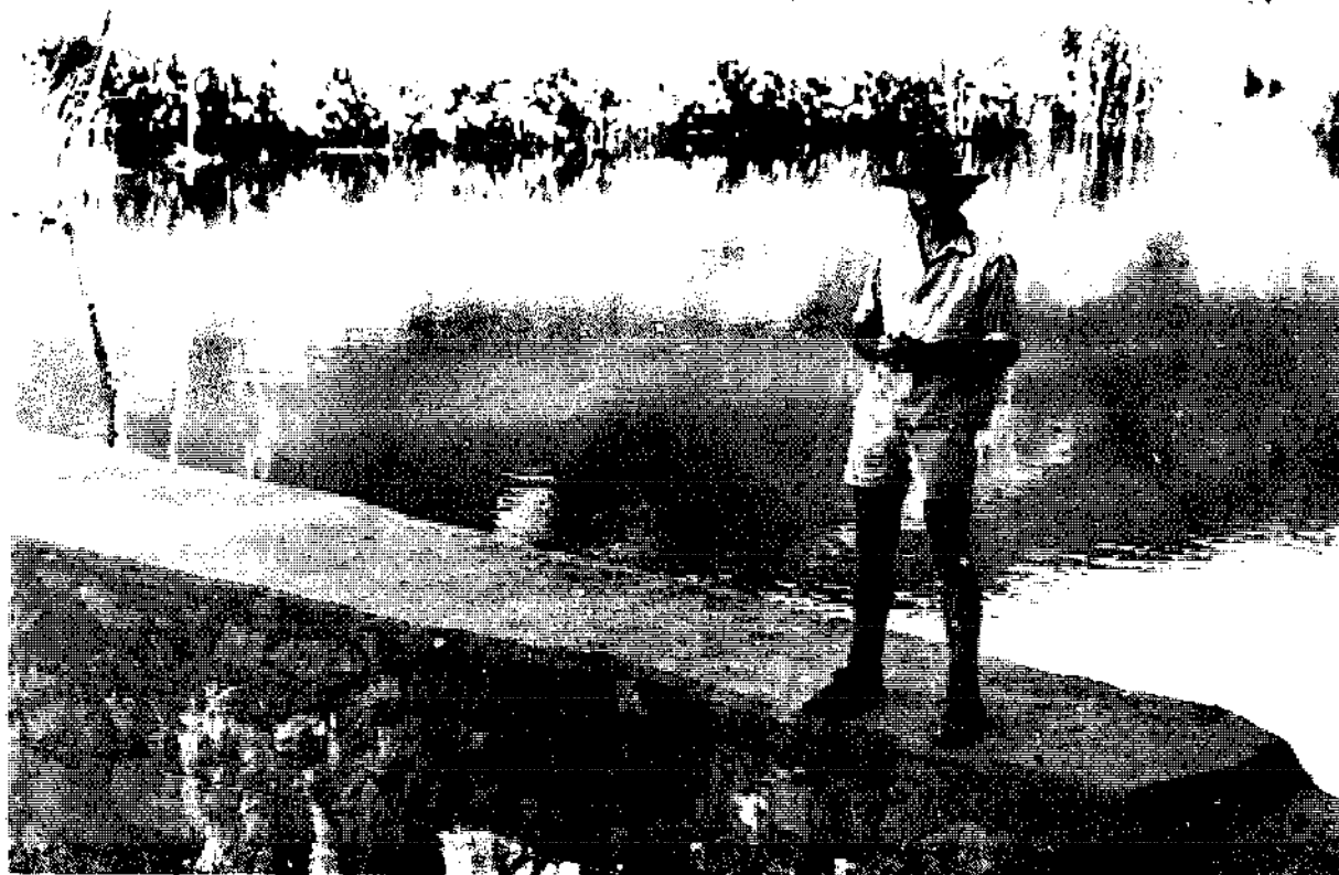
ALLEN JENKINS AT ULLUMPARA DAM IN A ROCK-WALLED VALLEY. DAM PLATE 5-5 PROVIDES AMPLE GARDEN WATER AT HEAD. MANY SUCH SITES ARE AVAILABLE IN DESERTS.
