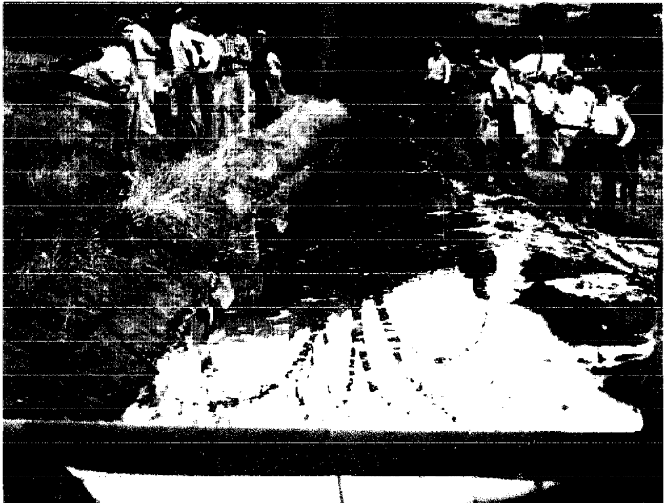
AT KIEWA (WALLACE FARM). IRRIGATION CHANNEL, BLOCKED WITH A CANVAS 'FLAG'. WATER SPILLS OVER INTO A CHISELLED FIELD.
