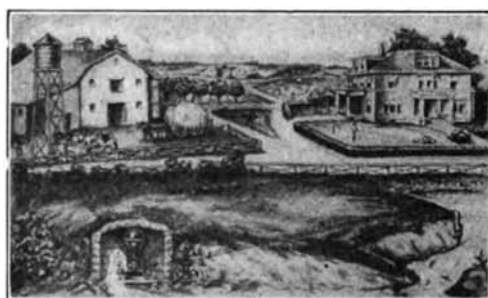
FIG. 220.—Hydraulic ram for filling tanks not more than 120 feet above the source of supply.
