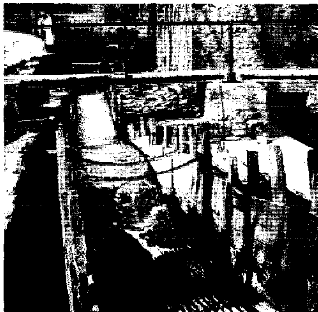
Fig 266 Gratings for catching eels in the outlet of a mill-pond in the Eifel/Germany. (Photo: G Jens.)
