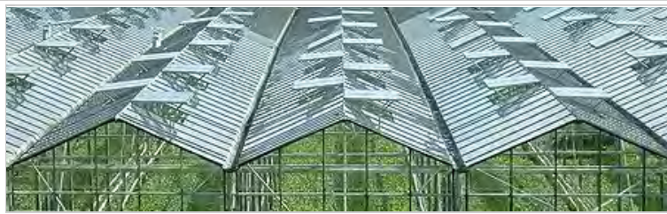
Greenhouses in the Westland region, Netherlands
