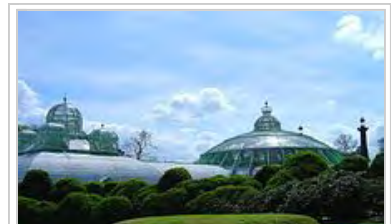
The Royal Greenhouses of Laeken, Brussels, Belgium. An example of 19th-century greenhouse architecture
