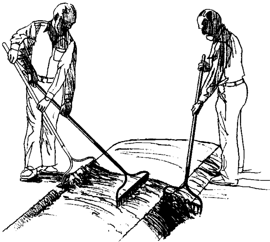
(Left) raking soil outward from inside for lip. (Right) raking soil up from side for lip.
