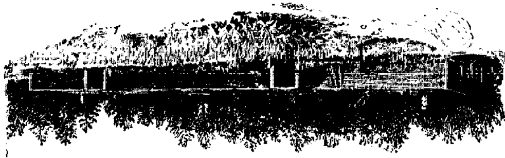
FIG. 207. Store-house for nursery stock, partly beneath the surface.
