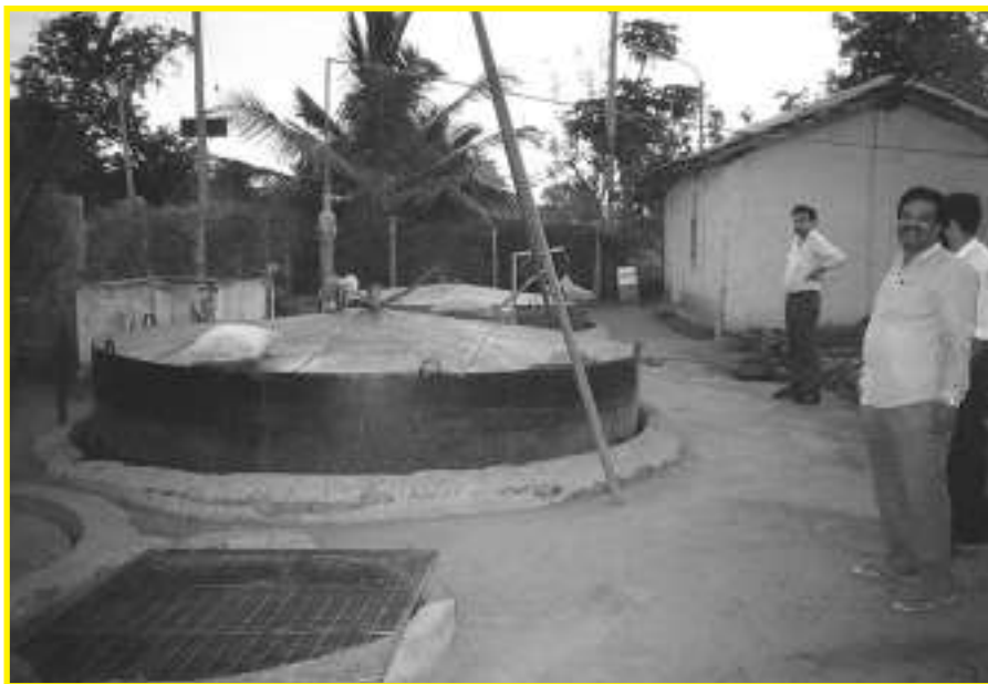
Anaerobic cattle dung digester producing biogas in the village of Pura, Karnataka State, India.
