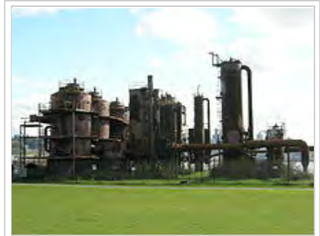
Gas Works Park, Seattle, preserves most of the equipment for making coal gas. The only such plant surviving in the United States.
