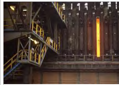
Coke oven at smokeless fuel plant, South Wales
