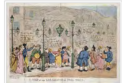
A Peep at the Gas-lights in Pall Mall: A contemporary caricature of Winsor's lighting of Pall Mall, by George Rowlandson (1809)
