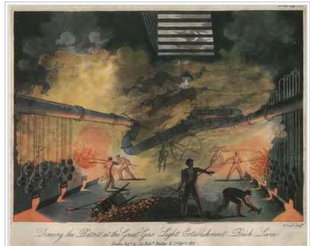
Drawing the retorts at the Great Gas Establishment, Brick Lane, from The Monthly Magazine (1821)
