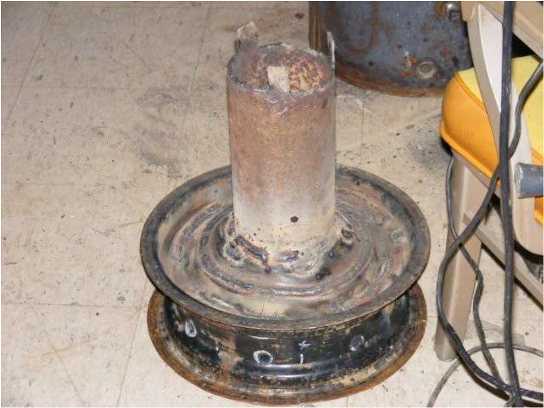
Rim completed. All holes welded closed. Pipe is 5" diameter 11.5" long. Rim is 14"
