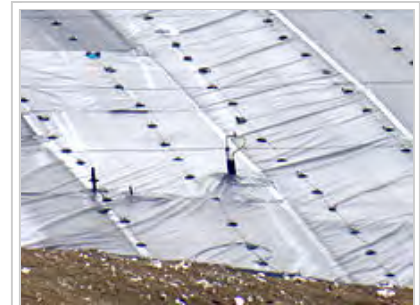
Landfill gas collection from capped landfill area
