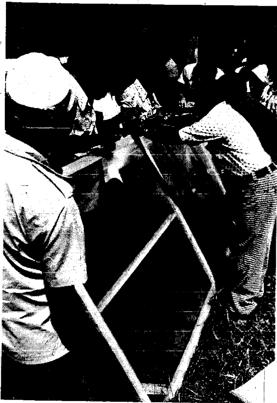
Making simple cover frame for Solar Dryer.
