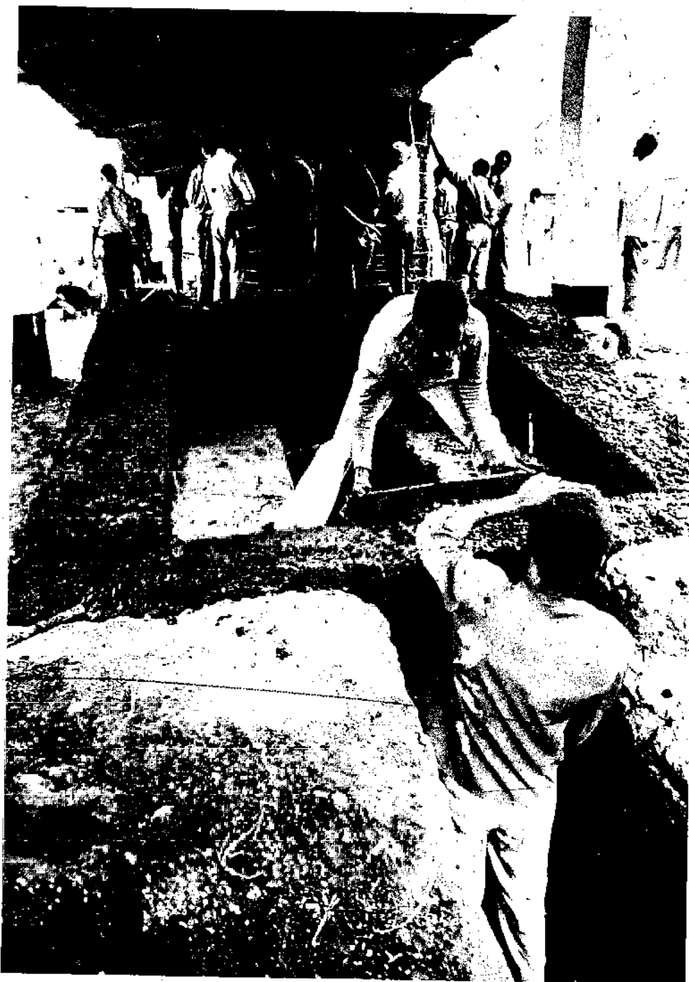
Photo – Erik Bentzen Mounting the dryer walls. (In the background is a nearly completed 4.5 ton cement stave silo.)
