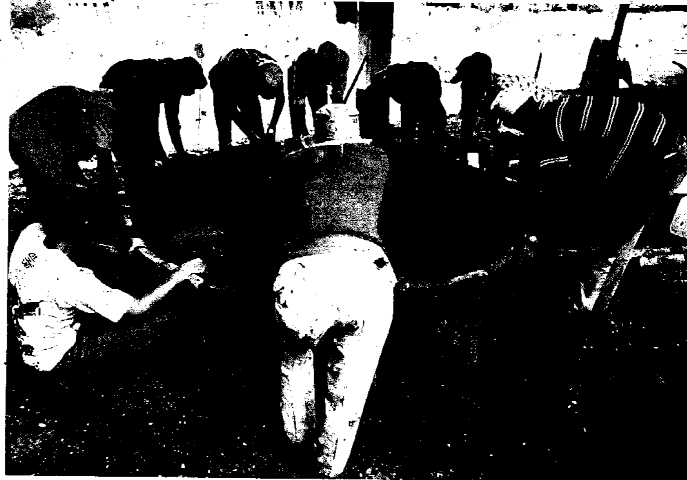
Form for floor slab consists of 29 large staves placed temporarily around outside foundation pillars in 111 cm radius. .
