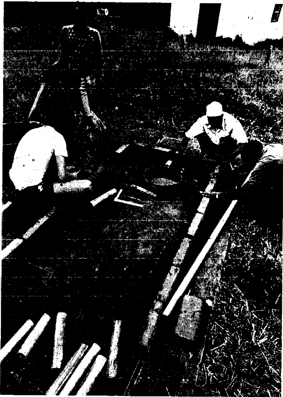
Early construction of Model 2 Solar Dryer
