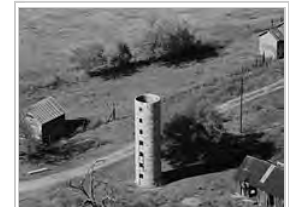
Silo 3.5 miles southeast of Blooming Grove Texas built c: 1900 by F. B. Cumpston. Used mainly for corn.
