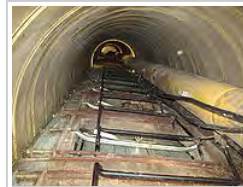
View of doors under shroud. Due to the limited space, the door hinge frame is also the ladder. On the right is the unloader power cable and yellow silage drop tube with removable access doors for insertion of the silage drop spout.
