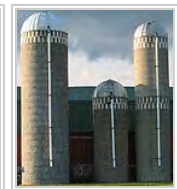
Small stave silos can be expanded upward. More hoops are added to strengthen the lower staves.
