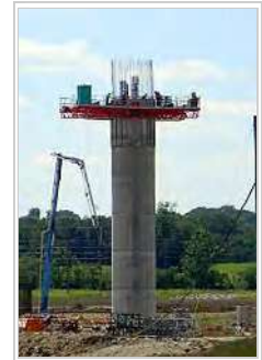
Coal silo under construction using aluminum concrete formwork
