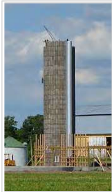
Concrete stave silo under construction in 2015
