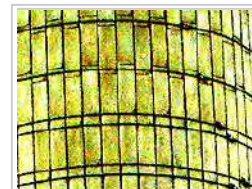
High contrast image showing the intermeshed concrete staves, and how the lower hoops are aligned over the stave edges.
