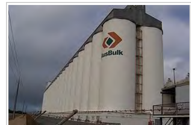
Grain elevators are composed of groups of grain silos such as these at Port Giles, South Australia.
