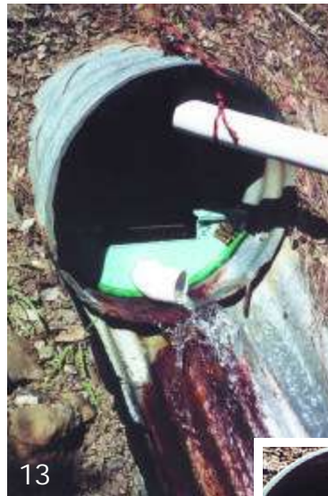
13. The diversion pipe from the culvert dam can be removed and tied off when not in use.
