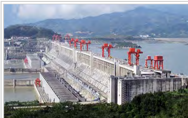
The Three Gorges Dam in Central China is the world's largest power producing facility of any kind.
