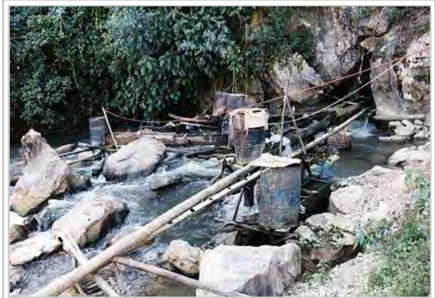
A micro-hydro facility in Vietnam
