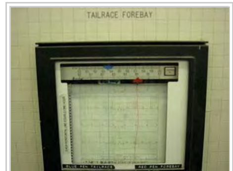
Measurement of the tailrace and forebay rates at the Limestone Generating Station in Manitoba, Canada.
