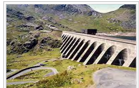
The Ffestiniog Power Station can generate 360 MW of electricity within 60 seconds of the demand arising.
