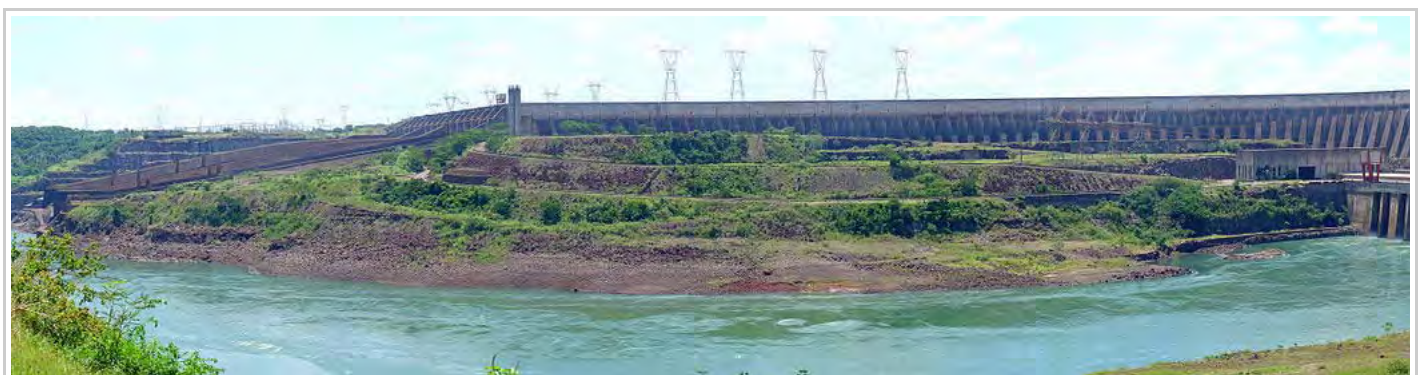
Panoramic view of the Itaipu Dam, with the spillways (closed at the time of the photo) on the left. In 1994, the American Society of Civil Engineers elected the Itaipu Dam as one of the seven modern Wonders of the World. [18]
