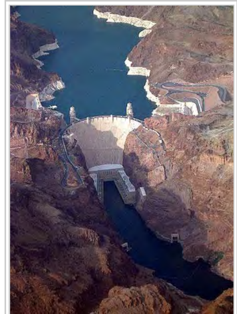
The Hoover Dam in the United States is a large conventional dammed-hydro facility, with an installed capacity of 2,080 MW.
