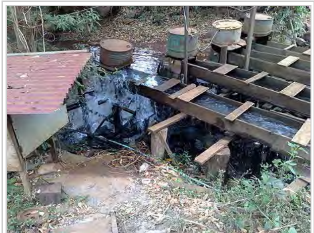
Pico hydroelectricity in Mondulkiri, Cambodia
