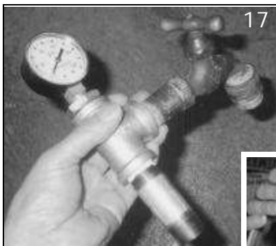
17. A pressure gauge and 3/4-inch drain valve are assembled, ready to be added to the pipe track.
