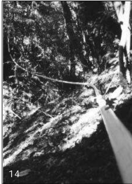
14. The pipe track stretches uphill and across a streambed.
