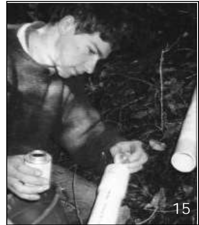
15. Jem Klein adds PVC glue before joining pipe sections.
