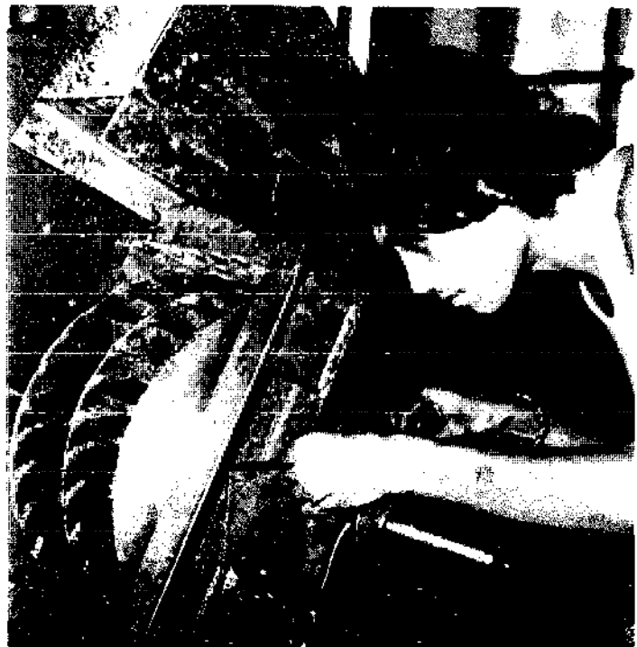
Fig. 27: T1 Assembly Work with Rotor, Flow- Regulator and Square Inlet (top) visible
