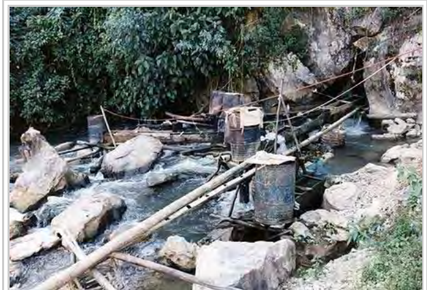
Micro hydro in northwest Vietnam
