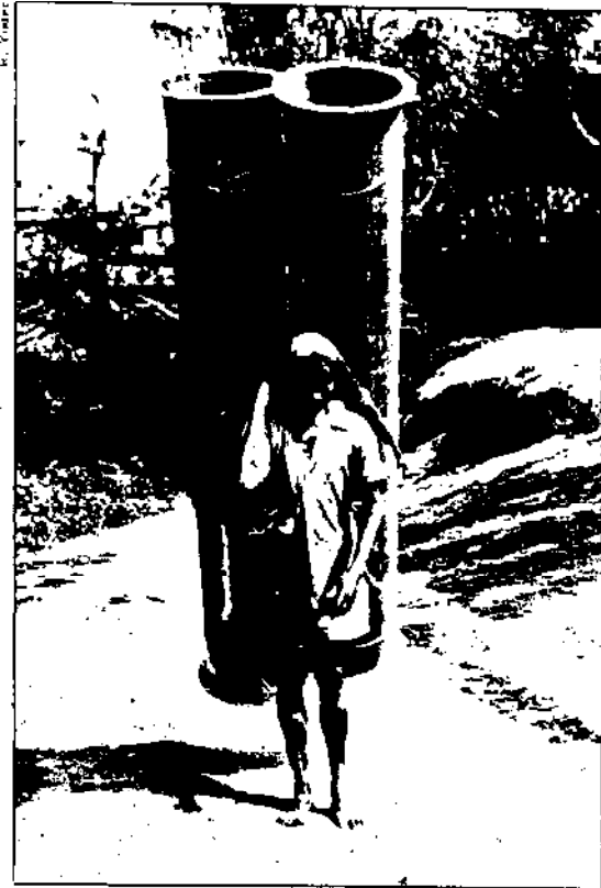
Fig. 27. After the site excavation has been completed and the equipment fabricated at Butwal, porters carry the necessary materials to the site. The two sections of penstock shown weigh about 100 kilograms.
