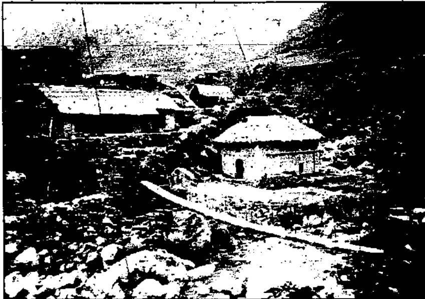
Fig. 1. A two-story mill house with the turbine and milling equipment on ground level and living quarters above is visible on the right. The penstock can be seen emerging from the forebay in the upper center of the figure.
