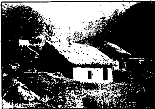
Fig. 21. A mill house with the owner's house in the background. The forebay and penstock can be seen at the left.
