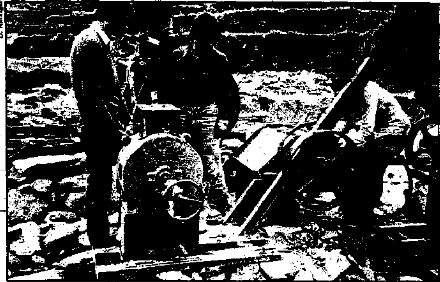
Fig. 17. The new turbines are mounted above the mill floor on a common mounting frame which is eventually set in concrete. Here the installation team is shown using a string to align the pulleys.
