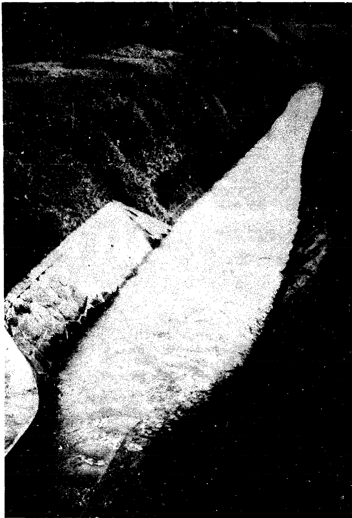
An unlined earth irrigation canal in Indonesia with masonry used only at points of potential erosion.
