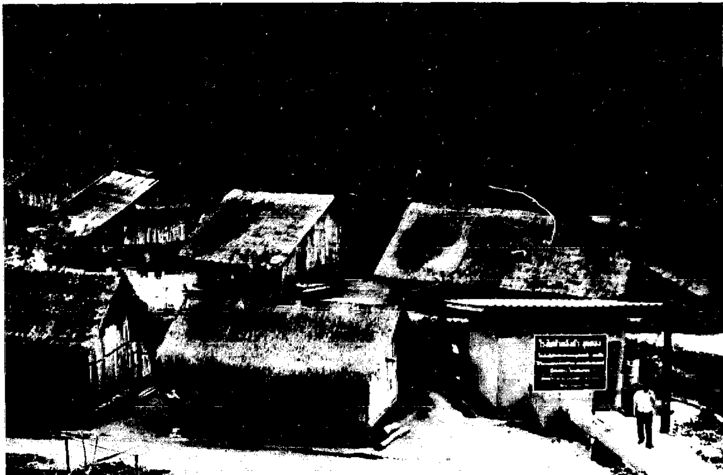
KHUN KHONG, THAILAND (12 kW) concrete power house and village houses wired for lights.
