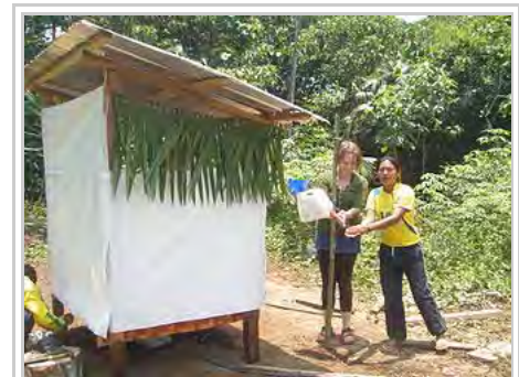
A tippy tap for handwashing after using a urine-diverting dry toilet in Pumpuentsa, Ecuador
