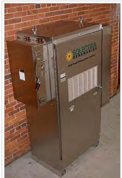
Three-phase grid-tie inverter for large solar panel systems
