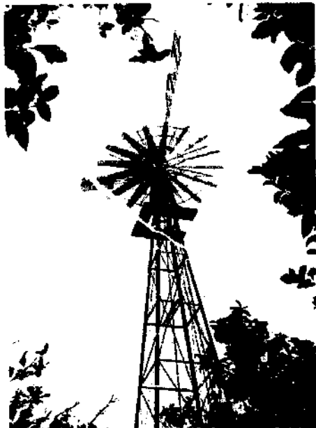
Prototype installed in Hammamet, Tunisia, irrigating an orchard.
