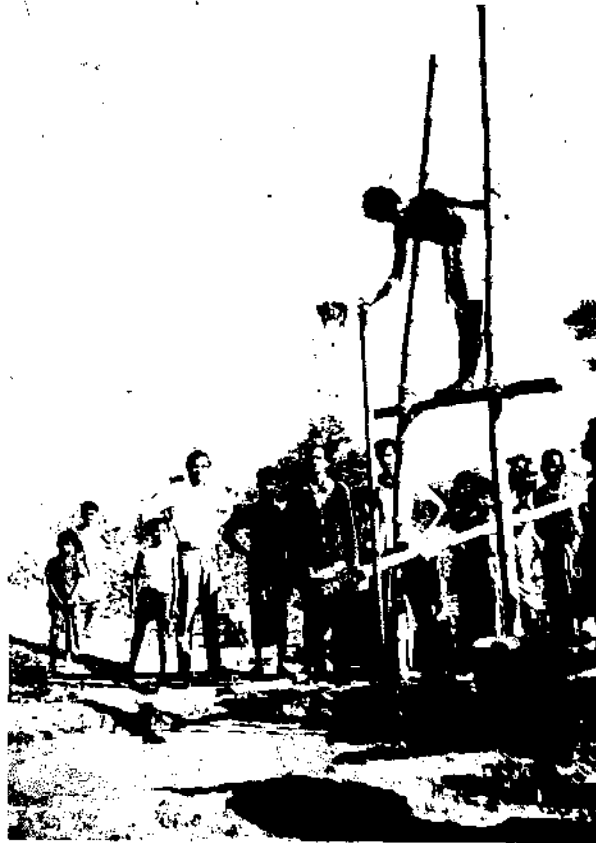
Fig. 18 4 inch diameter bamboo screen - bamboo strips wired to metal rings, then wound with coir rope
