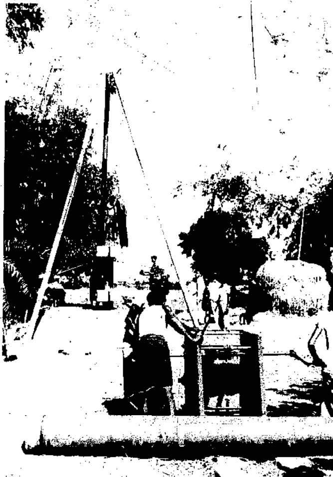
Bailing well with manpower
