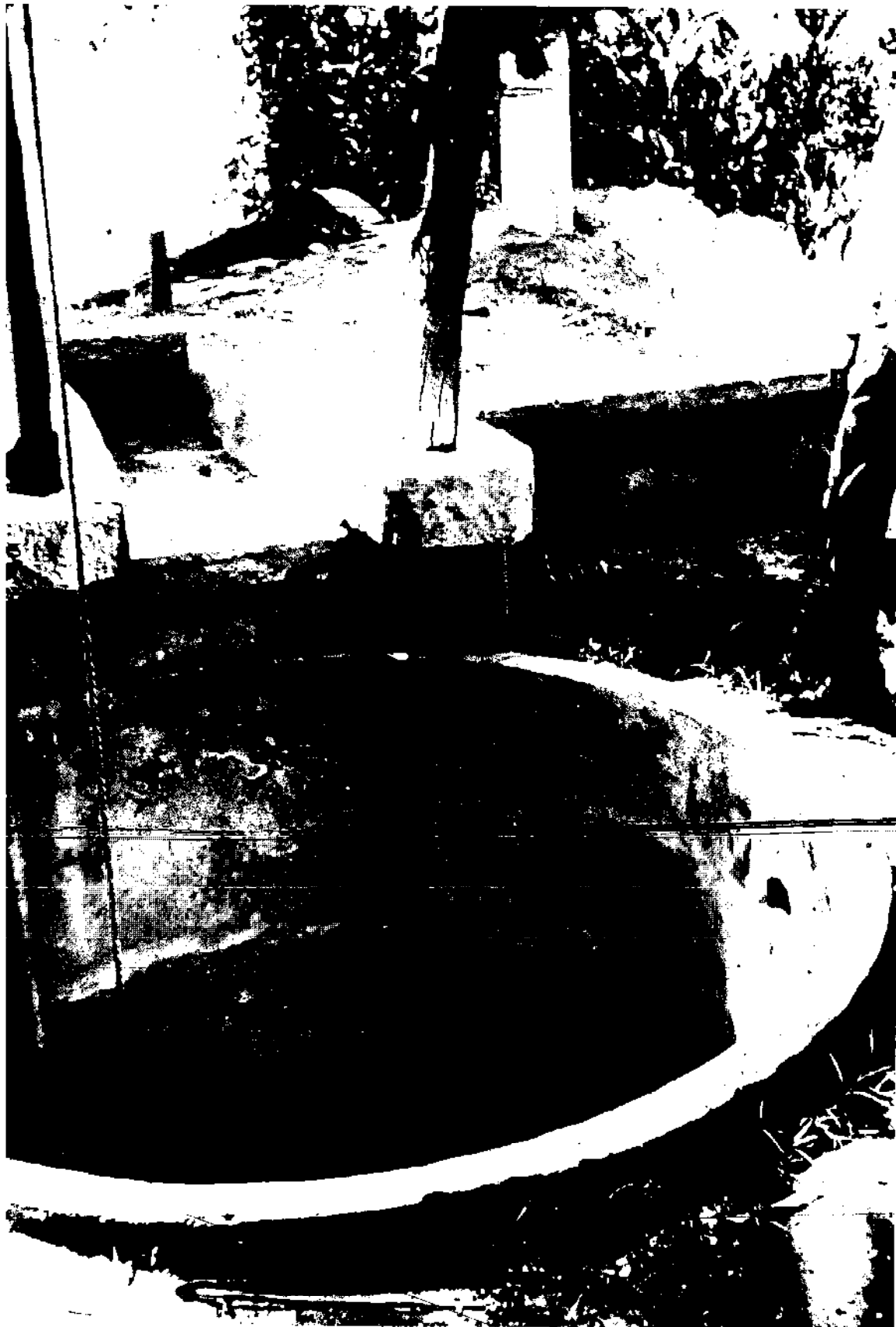
e diameter well equipped with stone channel to irrigation system into which skin buckets are emptied
