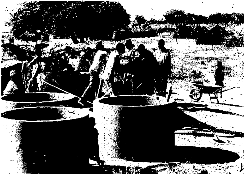
Fig. 51. Caisson sections made with commercially fabricated mould (Note perforations in surface to admit water)
