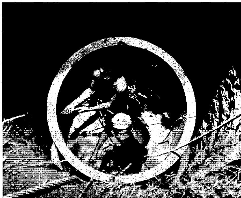
Fig. 45 Precast concrete caissons being set into a well excavated to the water table without lining
