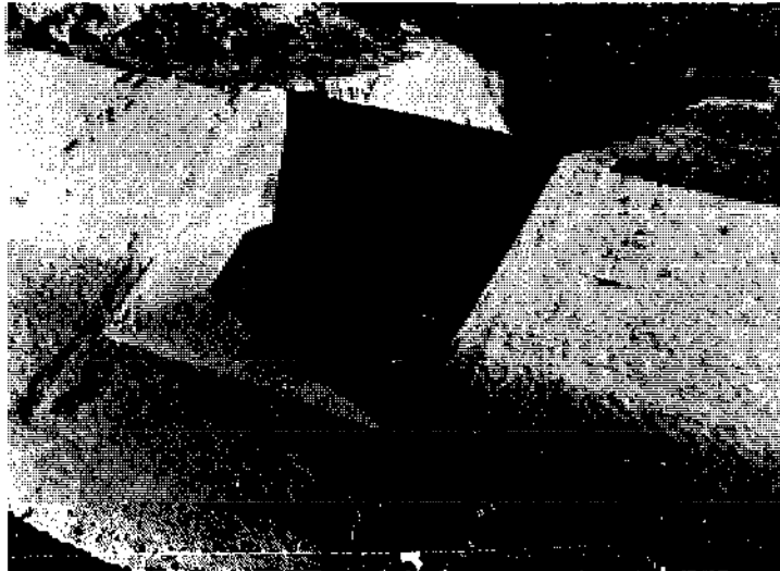
FIGURE 61. Weir-type outlet with flashboards in concrete-lined canal.
