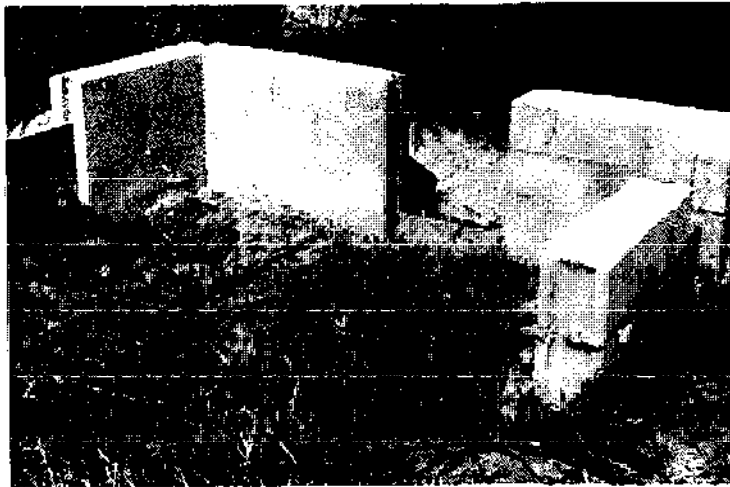
FIGURE 25. Control gate made of precast concrete blocks, in unlined canal.
