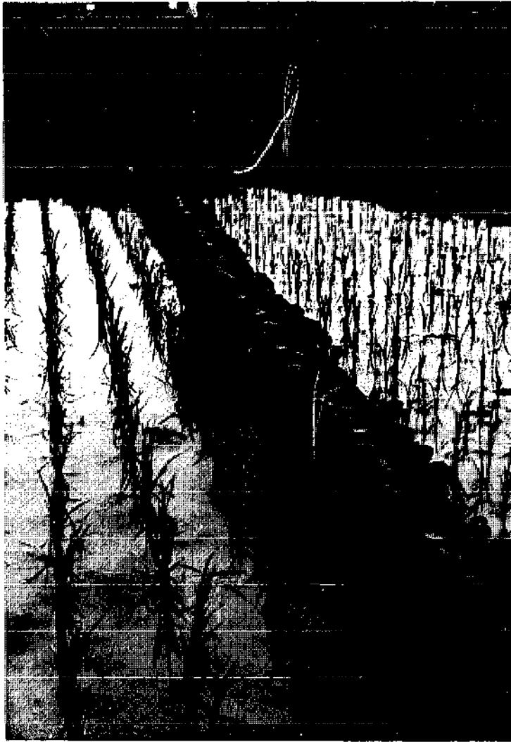
FIGURE 51. Earth levee between rice paddies constructed by hand labour. The levee also serves as a pathway for going in and out of the fields.
