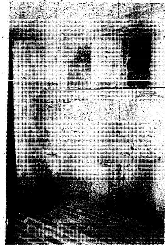
To support the drying trays bricks are projected at three levels on the two side walls.
