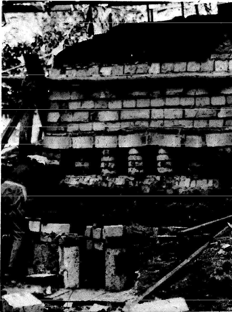
200. Work has started on the firemouth. The holes leading into the first chamber are clearly evident. The wood brace furnishes a buttress for the first chamber until the firemouth is complete.
