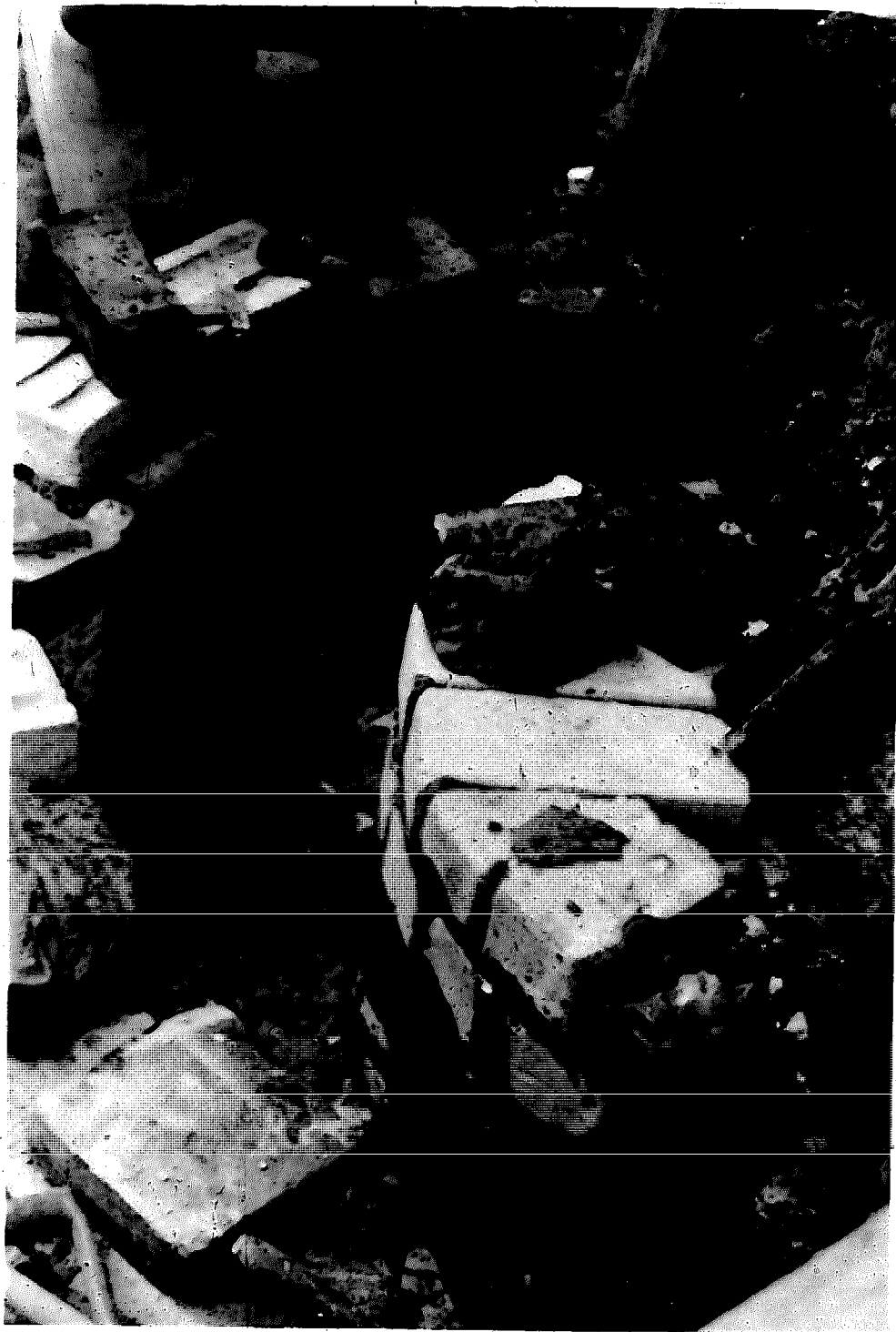
201. Construction of the firemouth. The level of the grate bars has been reached.
