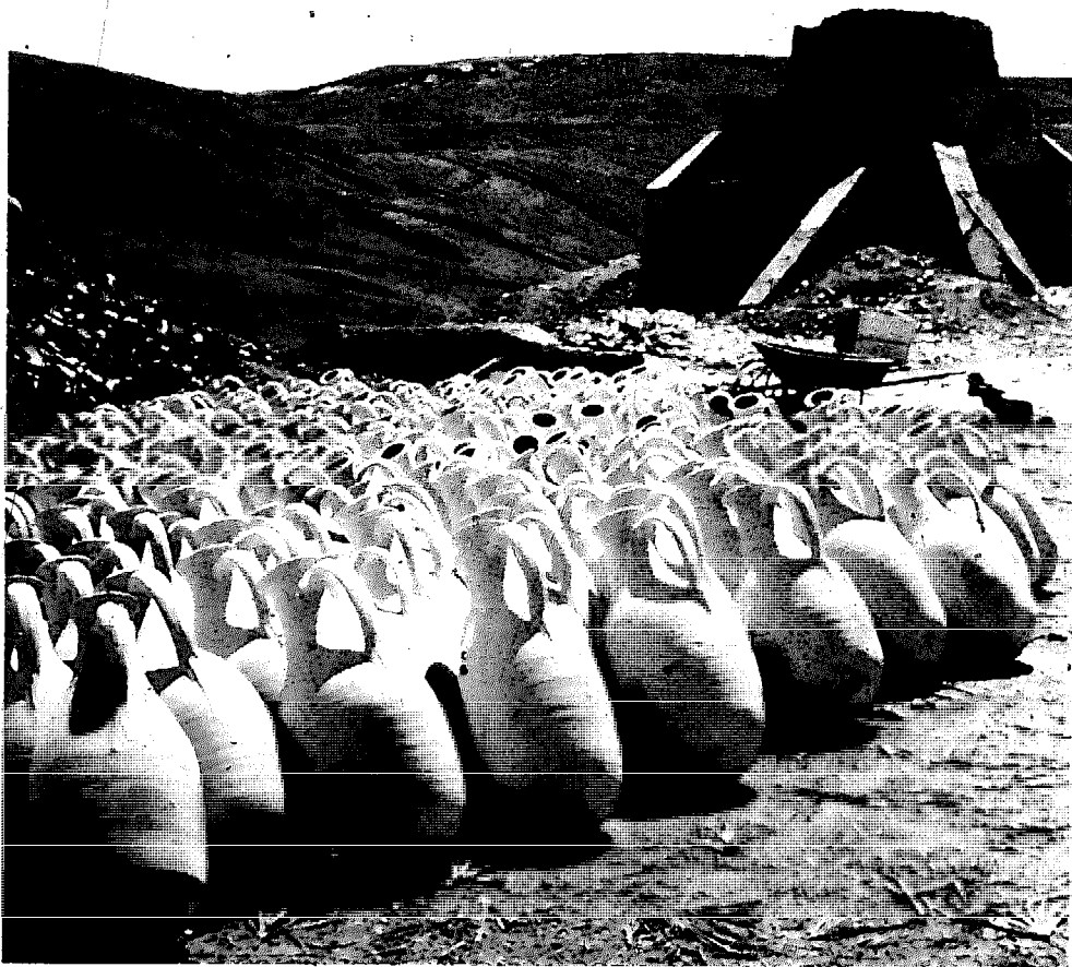
14. Large updraft kiln at Bab Tisra, Morocco. The walls of the cylindrical structure are heavily buttressed. Photo by Nan Sugar, courtesy of Craft Horizons.
