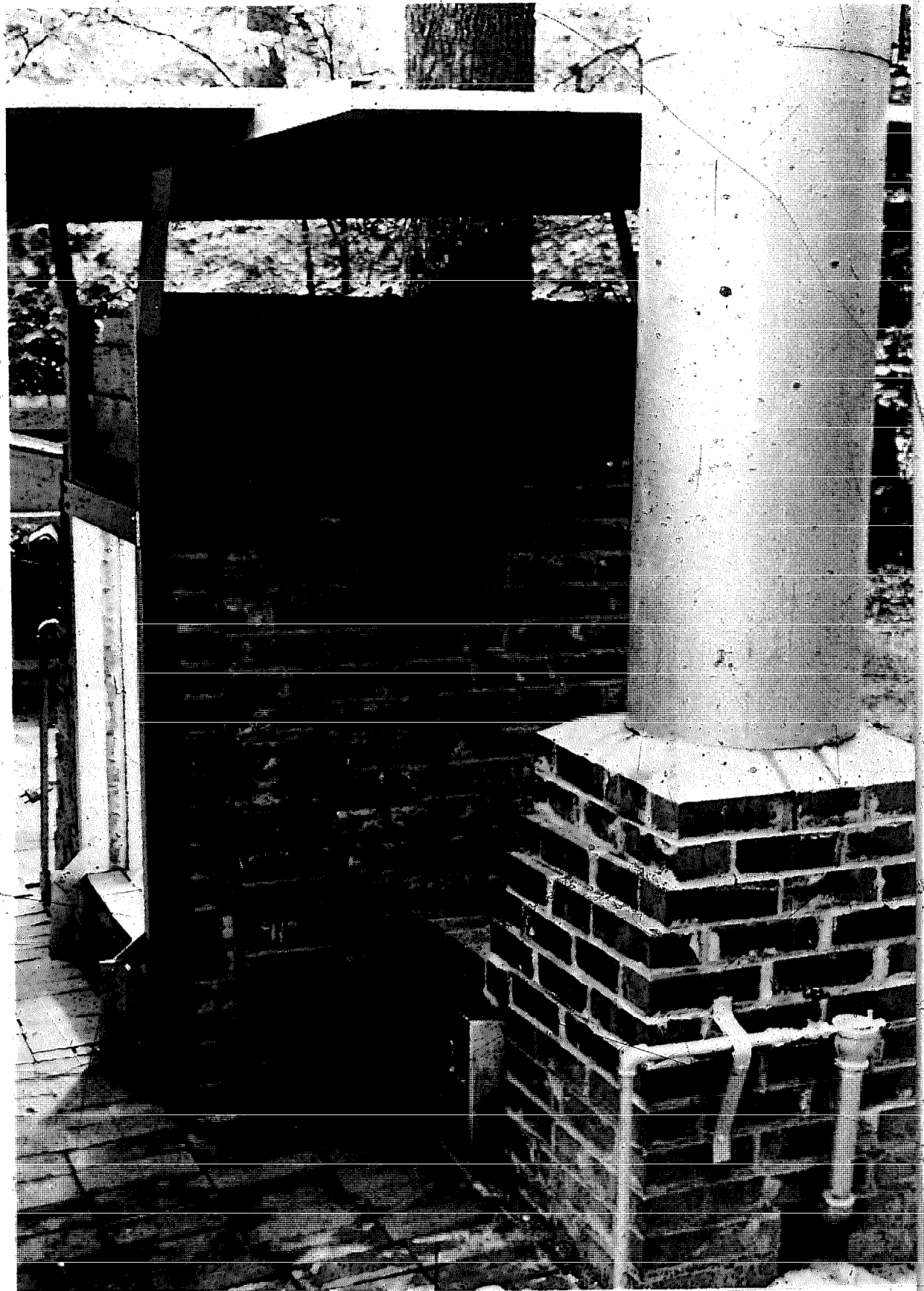
127. Stack. A burner is provided to warm the stack and induce a good draft for the early stages of firing.
