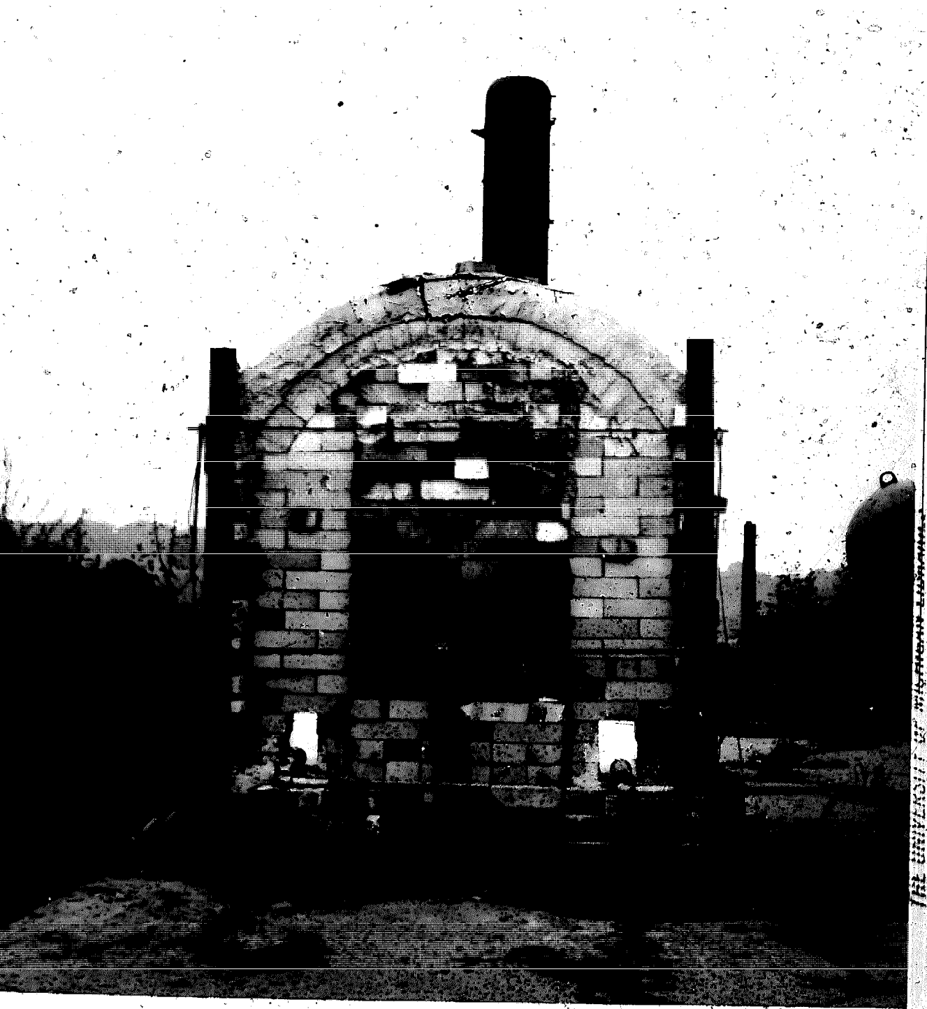
93. Don Reitz kiln firing on liquified petroleum gas. A second layer of brick has been added to the side walls and arch.
