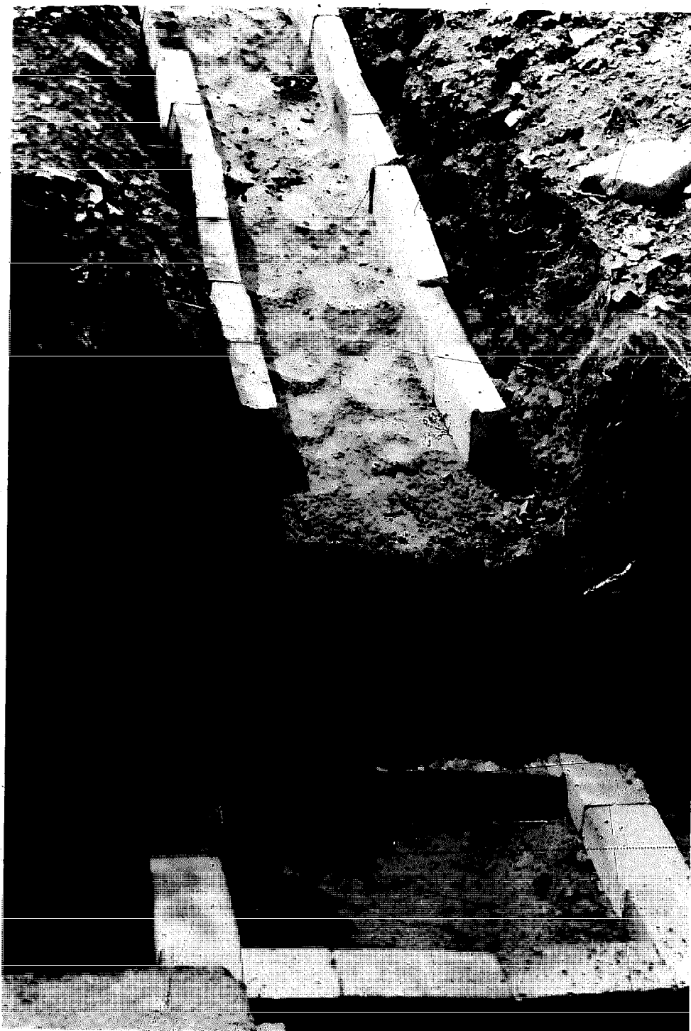
177. Starting the walls of the trench and the firebox. The bricks are placed directly on the ground.
