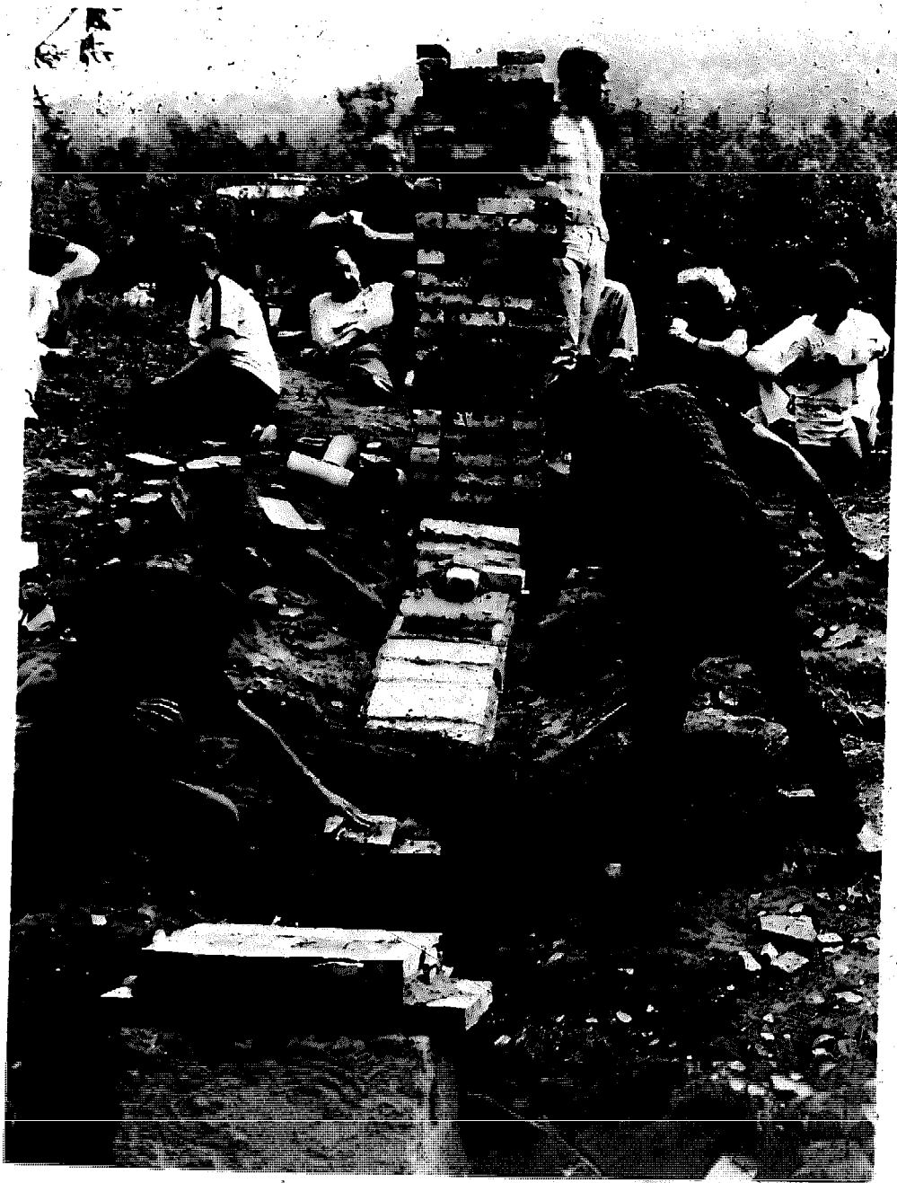
181. The top of the kiln is covered over with dirt. Photo by Ed Custer.
