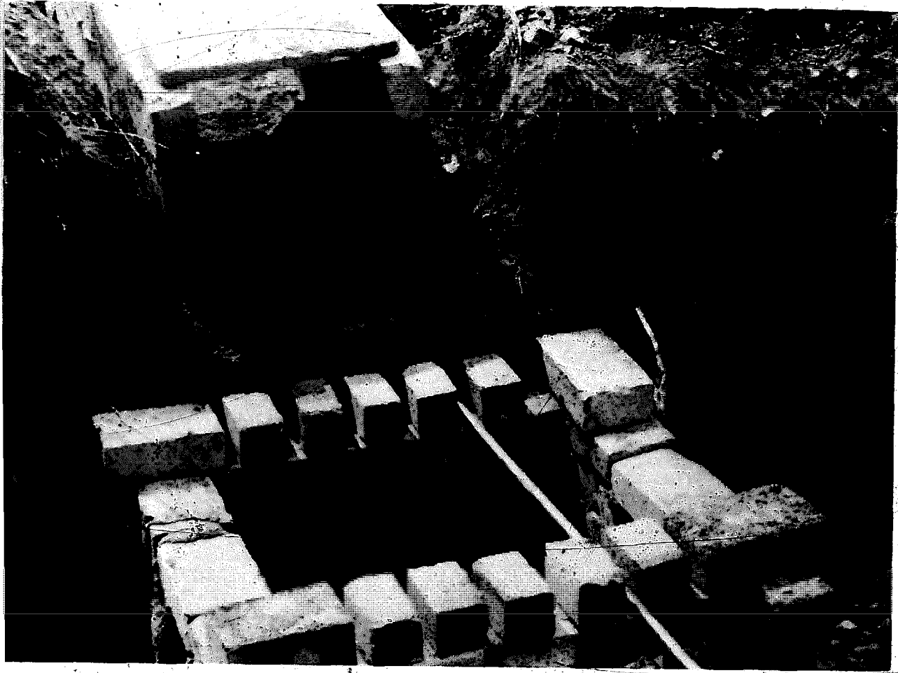
178. Construction of the firebox and ware chamber. The notches will hold the metal grate rods.
