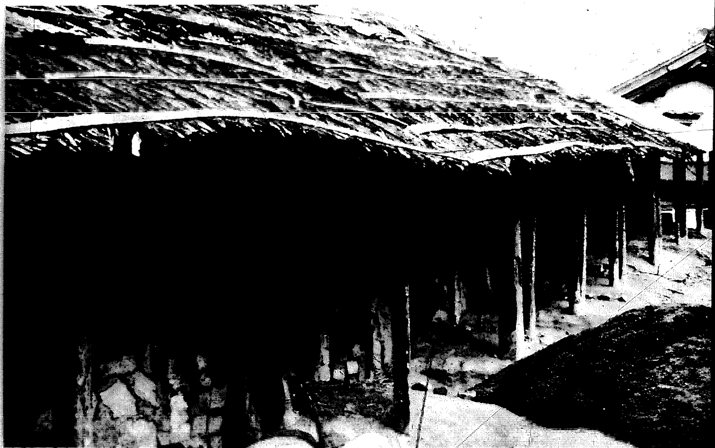
26. Kiln at Ryomonji, in southern Japan. The kiln shed is roofed with cypress bark.
