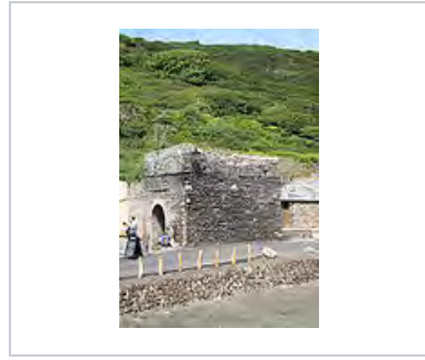
Old lime kiln, Boscastle, Cornwall.
