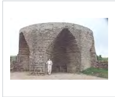
Large 19th-century single limekiln at Crindledykes near Housesteads Northumbria.
