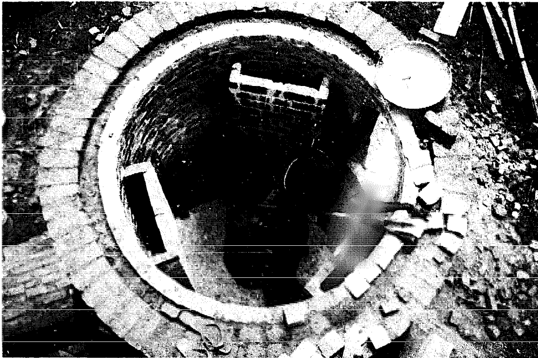
Fig. 2-101: Starting the dome of the Bujora kiln. Note the insulating loose layer between the inner firebrick lining and the outer wall. The bagwalls proved to be too high and were later cut in half.
