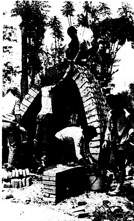
Fig. 2-106: Each row of arch bricks is completed at a time. Nepal.
