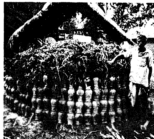
Fig. 2-8: Semi-permanent up-draught kiln in Rajshahi, Bangladesh. After smoking a layer of straw and mud is plastered on the outside.
