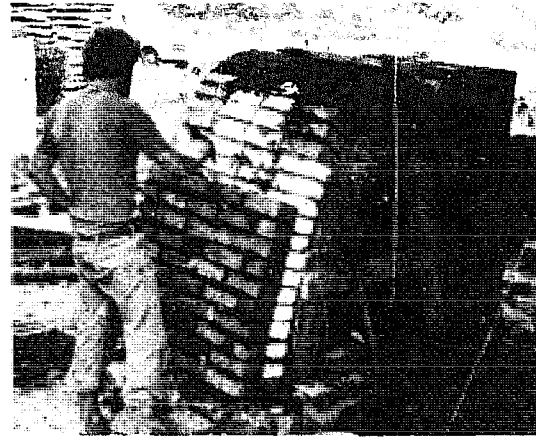
Fig. 2-104: Catenary arch under construction. Singisi, Tanzania.
