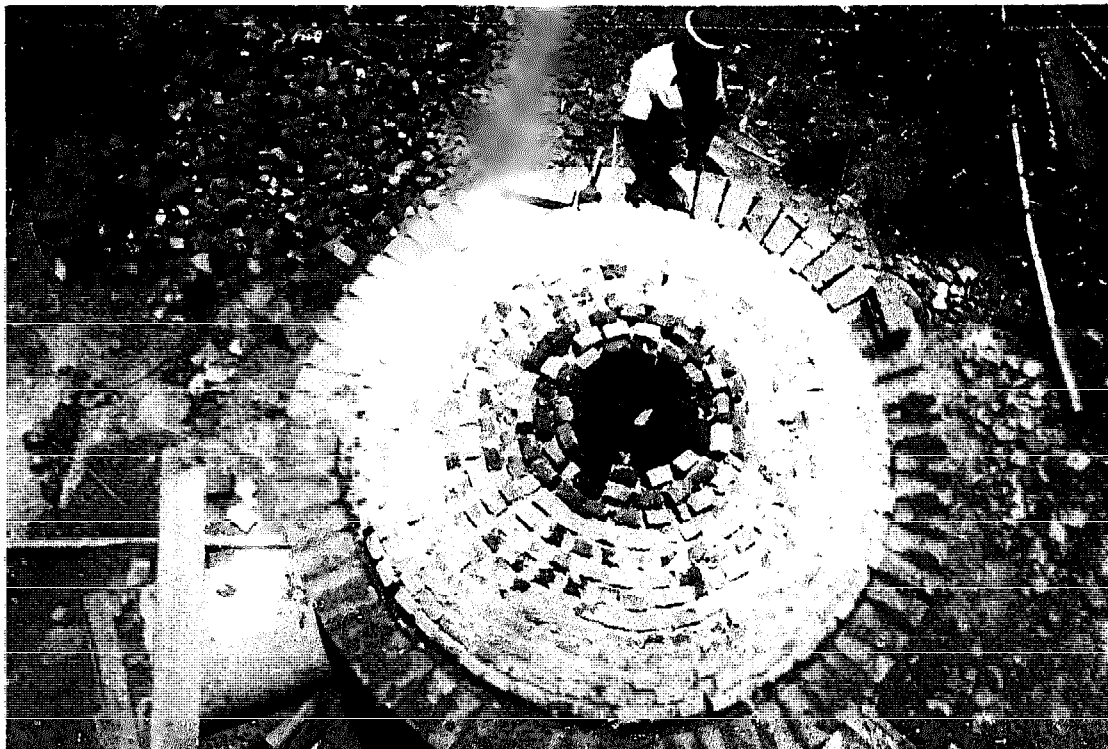
Fig. 2-102: Only a few courses are still to be laid and each brick has to be cut to size.
