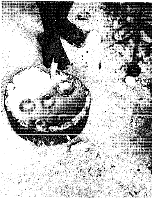
Fig. 2-138: Drawing a test cup through the spyhole with the help of an iron rod
