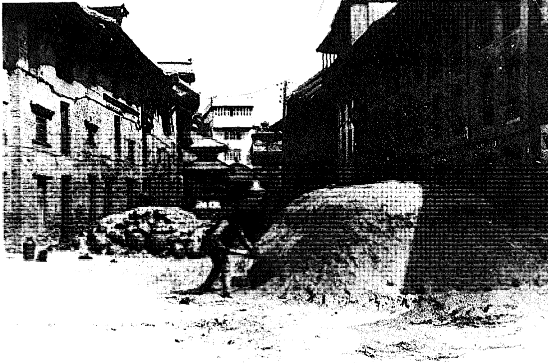
Fig. 2-4: Straw-fired kiln in Thimi, Nepal
