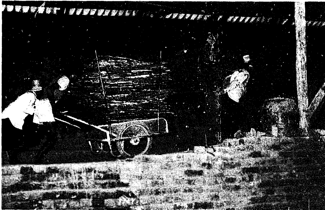
Fig. 2-41: Split bamboo sticks are dried on top of a sloping tube kiln.
