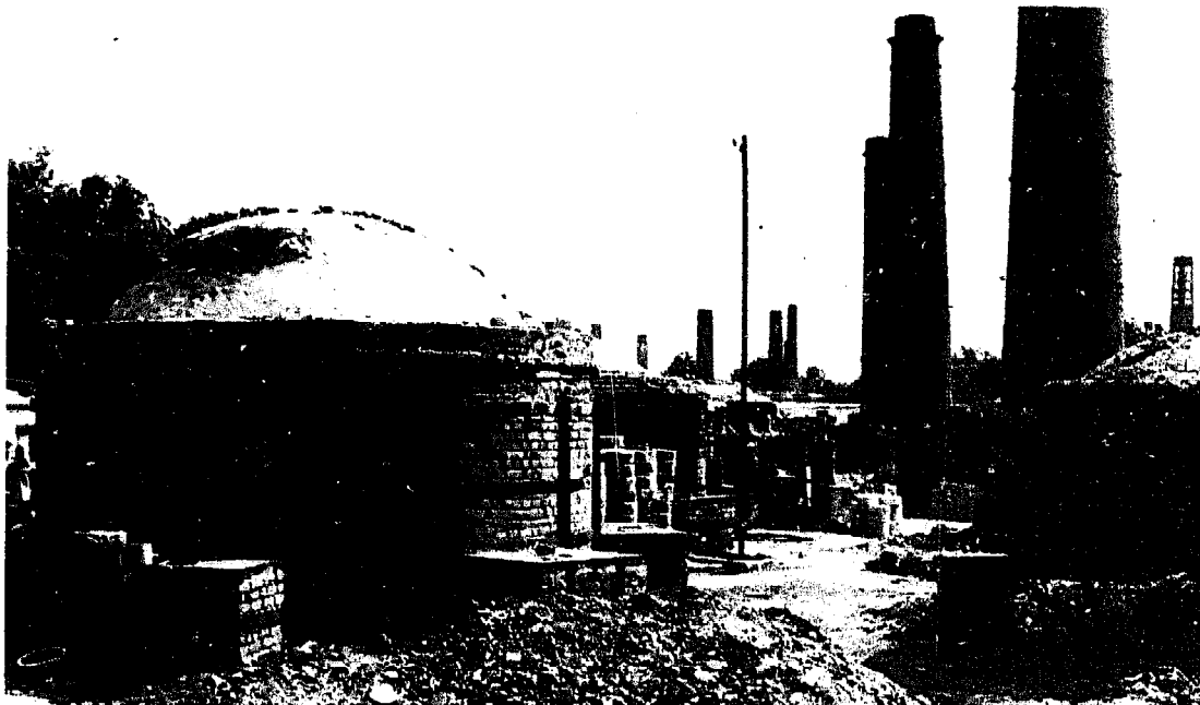
Fig. 2-18: Circular coal-fired down-draught kiln. Khurja, India.
