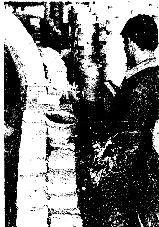
Fig. 2-86: Stretcher courses in a Chinese-type tube kiln
