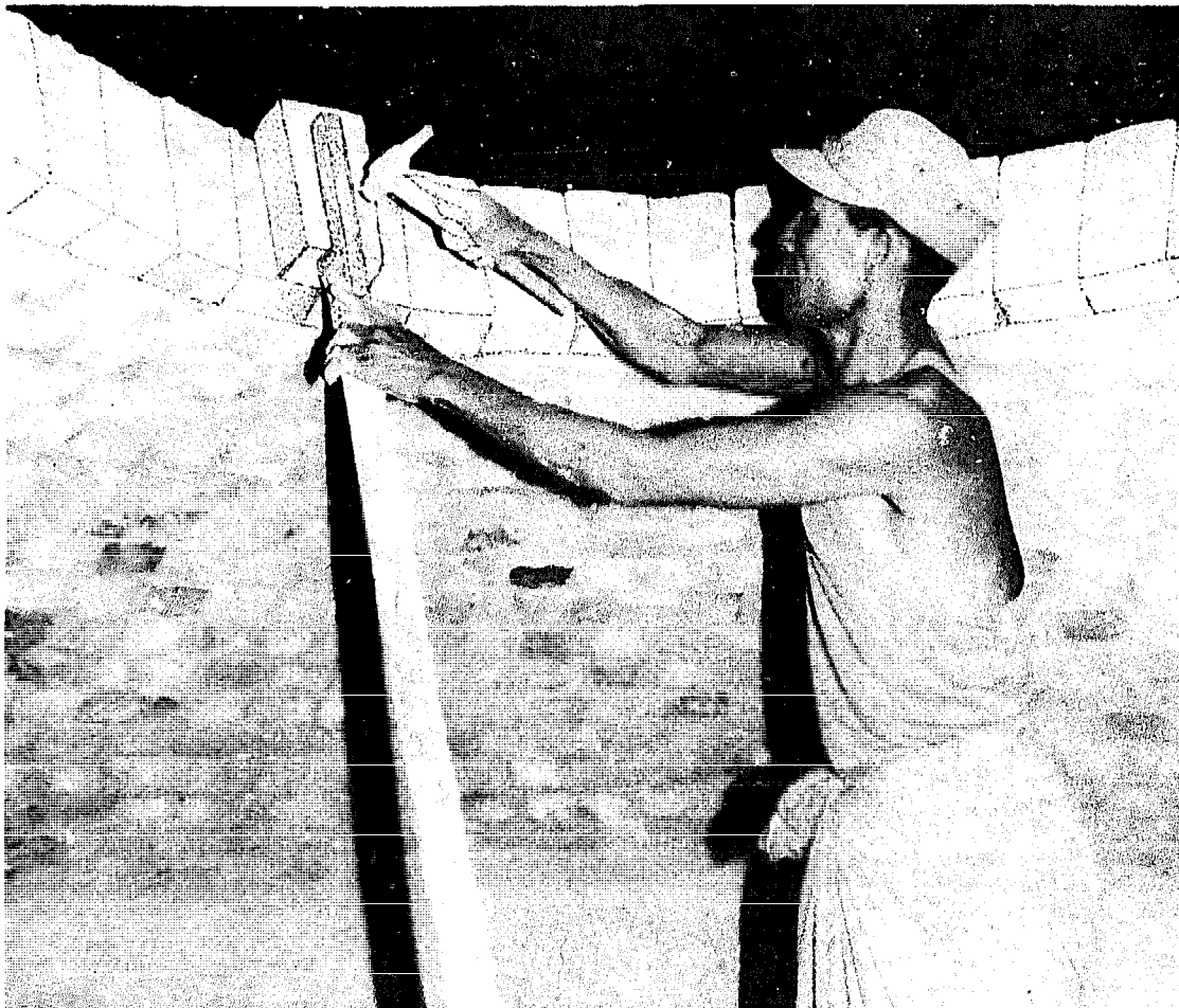
Fig. 2-98: Construction of a dome
