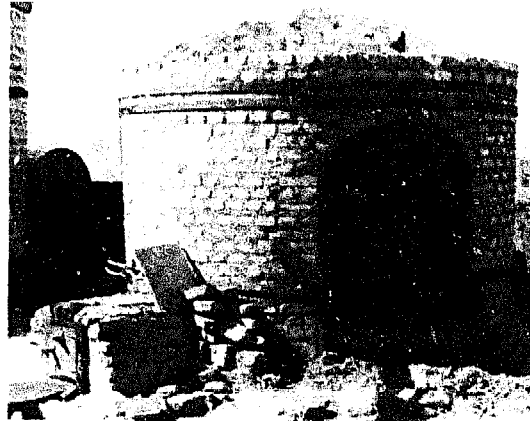
Fig. 2-21: First chamber of Bujora kiln. Water and oil pipes lead to the three fireboxes.
