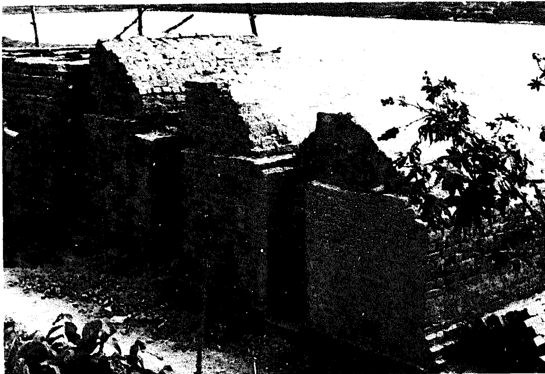
Fig. 2-31: Three-chambered wood-fired kiln under construction. The firebox to the right and the chimney at the other end are not yet ready. Champaknagar, Bangladesh.
