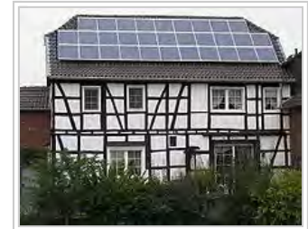
Rooftop PV on half-timbered house
