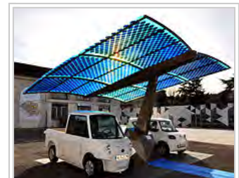
Photovoltaic SUDI shade is an autonomous and mobile station in France (developed by Hervé Thermique and Solutions Composites ( http://www.solutionscomposcat4-501.html )) that provides energy for electric vehicles using solar energy.
