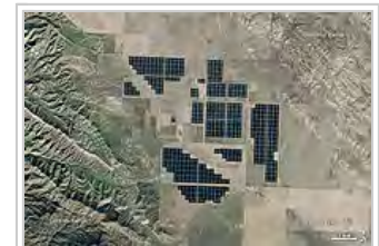
Satellite image of the Topaz Solar Farm
