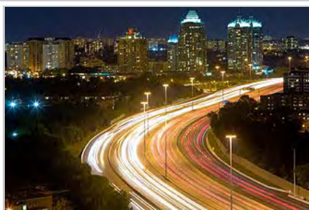
High mast lighting along Highway 401 in Ontario, Canada.
