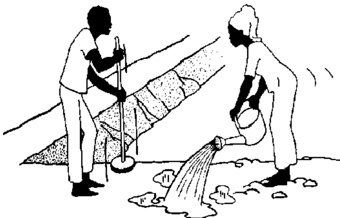
Figure 32: Compacting the dike (Viveen et al., 1985).
