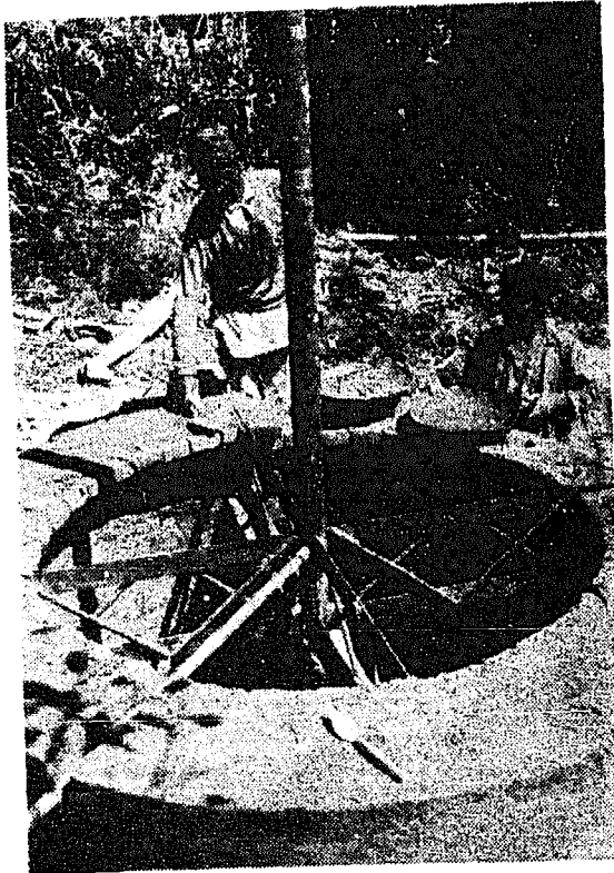
This picture shows the dividing wall in the pit, the fixture of the vertical guide pipe, and the gas outlet.
