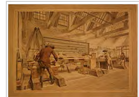
Exact drawing made with camera obscura of horizontal boring machine by Jan Verbruggen in Woolwich Royal Brass Foundry approx 1778 (drawing 47 out of set of 50 drawings)
