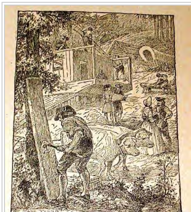
PIONEER SETTLERS BUILDING ADVENTURE GALLEY ON THE YOUGHIOGHENY
