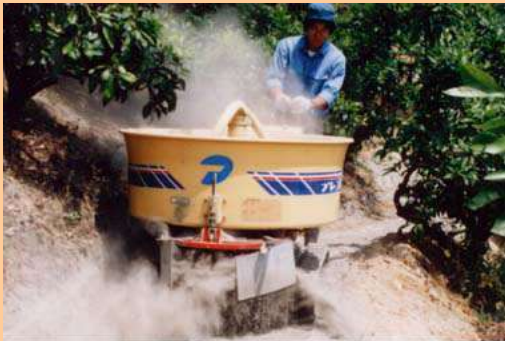
Fig.2. Construction process of farm path
