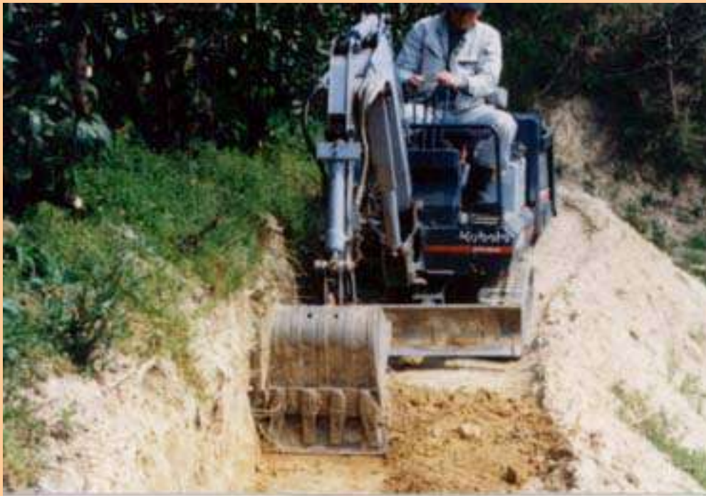
(1) Digging out using a small back hoe
