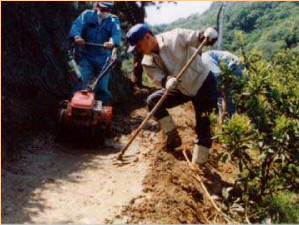
Fig.2. Construction process of farm path
