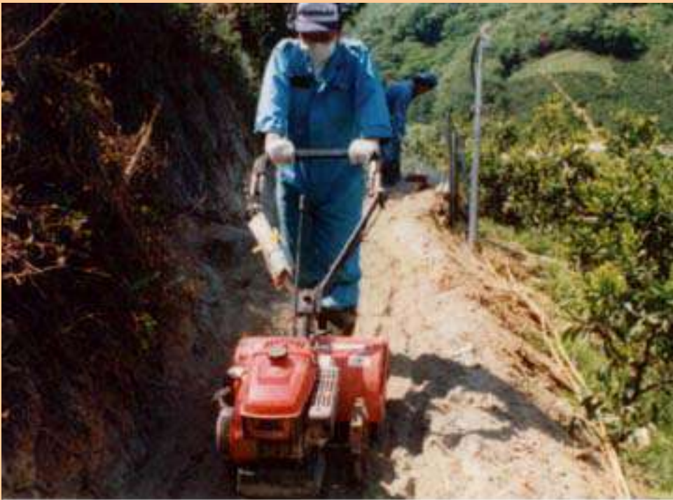
Fig.2. Construction process of farm path
