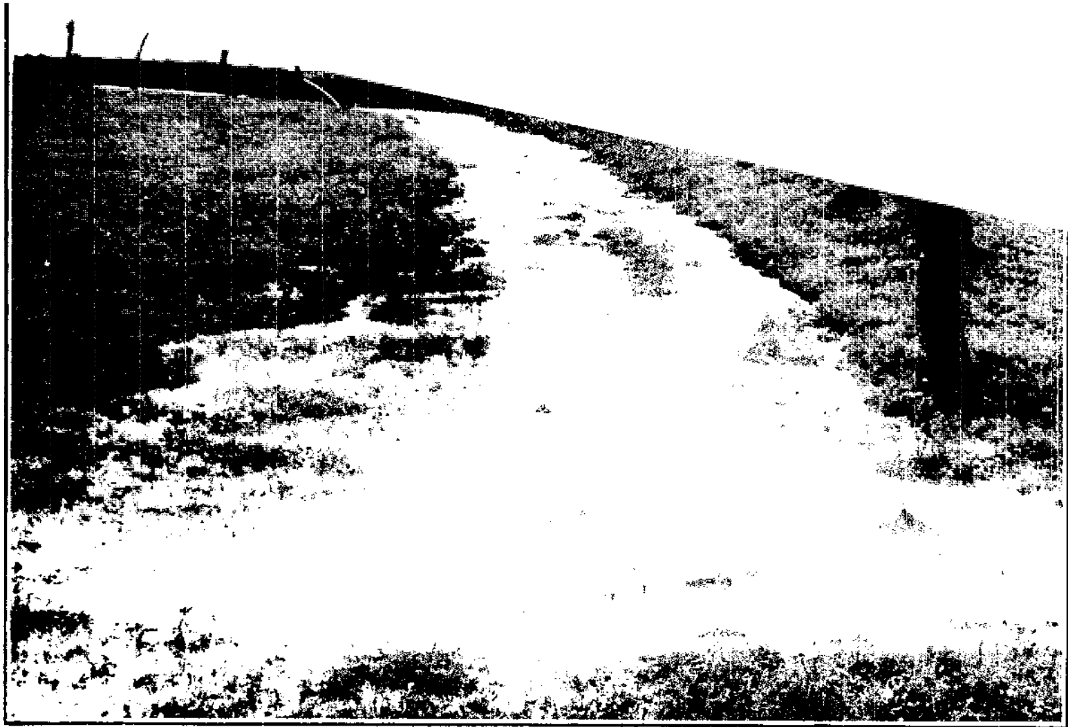
FIG. 132. An inch of rain fell in Haskill Co., Oklahoma, in half an hour. A terrace pours its surplus into a grassed channel that will not erode, and spreads the water over a pasture. (Photo Hulnagle, U. S. Soil Conservation Service.)
