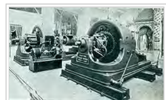
Westinghouse alternating current polyphase generators on display at the 1893 World's Fair in Chicago, part of their "Tesla Poly-phase System". Such polyphase innovations revolutionized transmission
