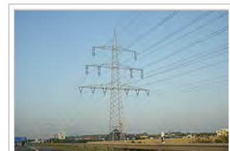
Four-circuit, two-voltage power transmission line; "Bundled" 2-ways
