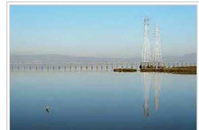
Power lines in the San Francisco Bay Area
