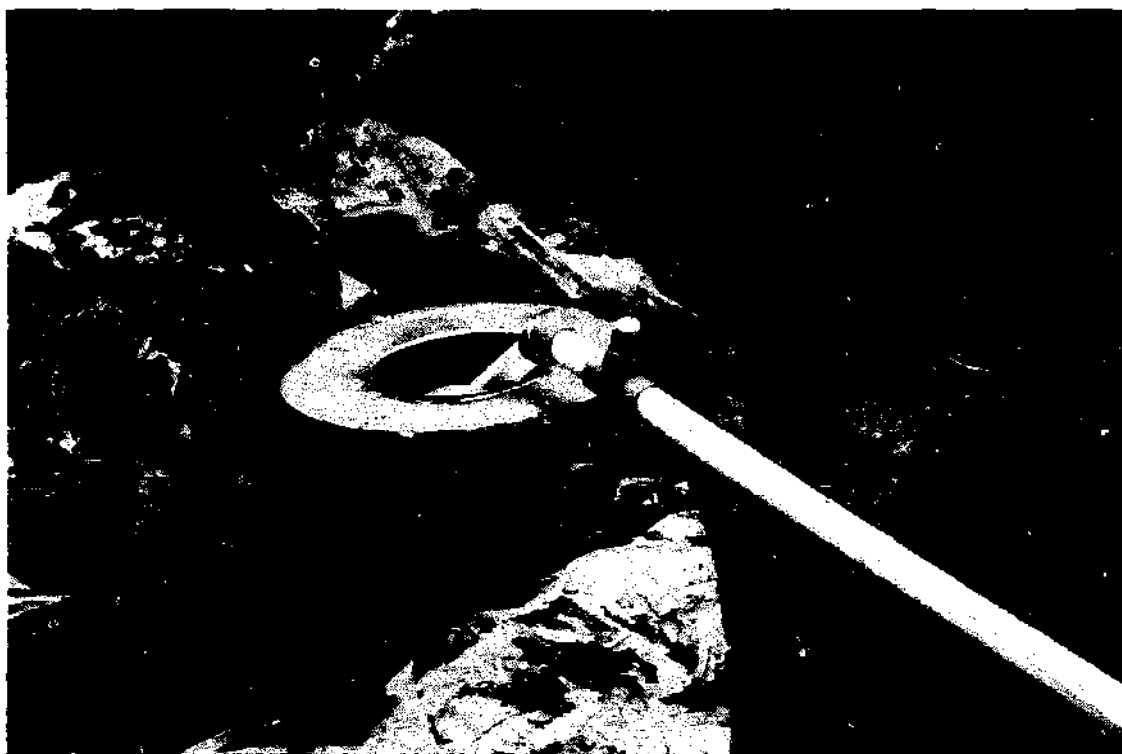
FIGURE 19 A 3-in. (7.6-cm) PVC pipeline carrying 130 gal of water per minute (492 l/min) over a distance of 2,500 ft (762 m), developing a net head of 400 ft (122 m), and producing 5 kW of electrical energy (see the nomograph in Figure 25). (Photograph courtesy of Independent Power Developers, Inc., Sand Point, Idaho)
