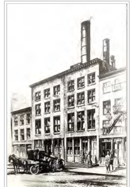
A sketch of the Pearl Street Station, the first steam-powered electric power station in New York City
