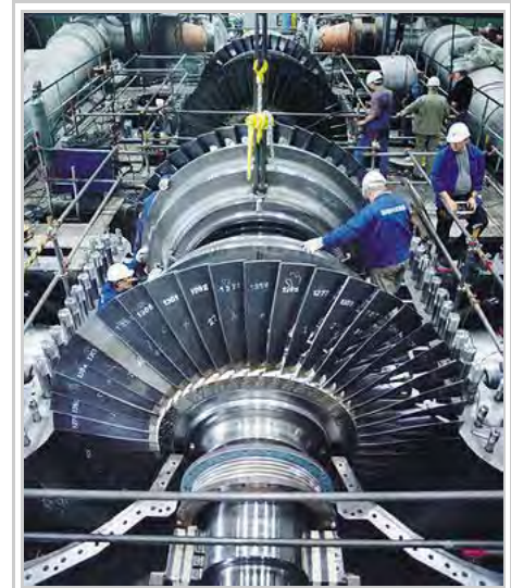
A steam turbine used to provide electric power.
